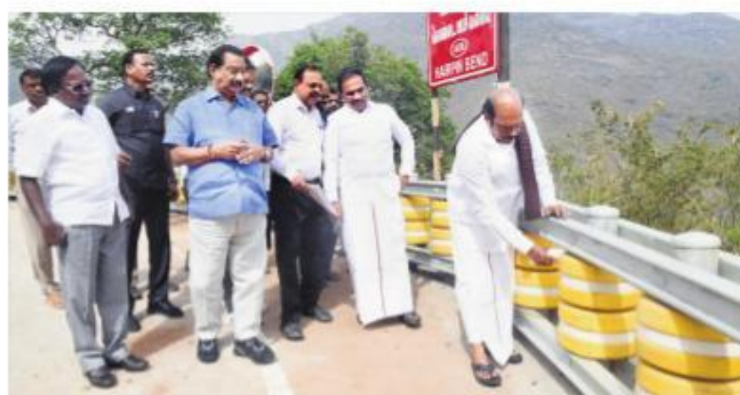
Highways minister EV Velu checks out a newly installed roller barrier | EXPRESS
